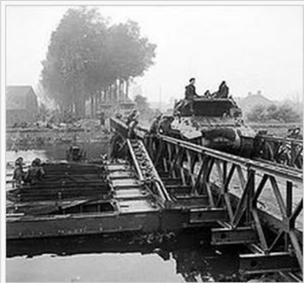
British M10 tank destroyers using a Bailey bridge to cross a canal near Lille St. Hubert, Belgium (September 1944). The bridge is supported by pontons
